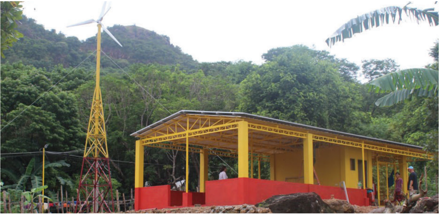
Powerhouse and wind turbine in Brgy. Decabaitot, Linapacan, Palawan
